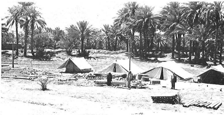
Typical temporary line construction depot
