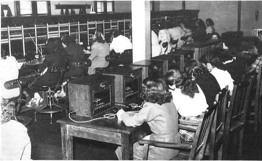
Baghdad automanual switchboard with enquiry positions in foreground
