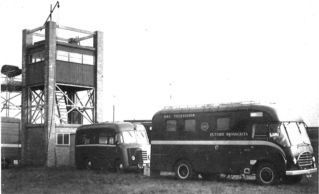
Mobile control room and Post Office vehicle at Becher's Brook
