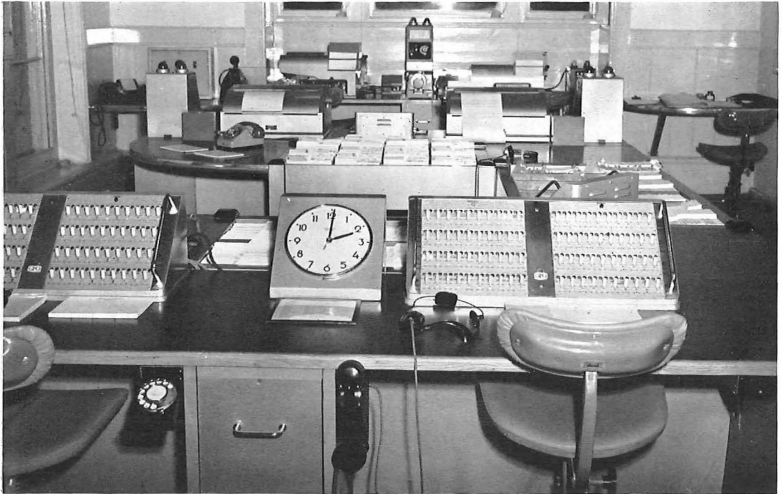
Surrey Fire Brigade, Reigate control room
