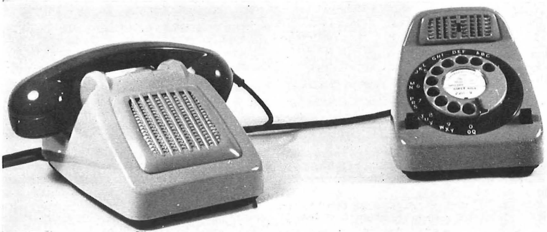
Fig. 5: One of the suggested models of the proposed loud-speaking telephone
