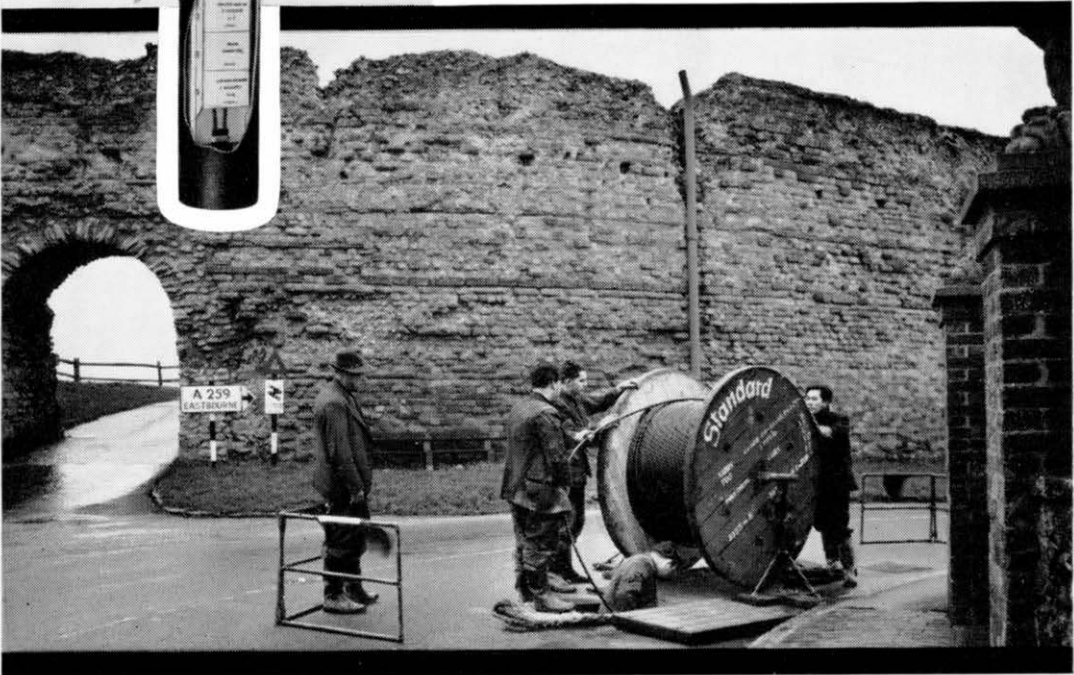
S.T.C. all-transistor buried repeater
