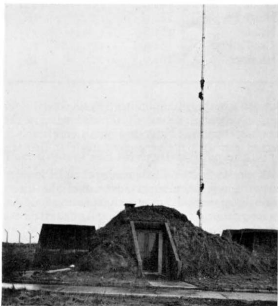
Fig. 1 : Niton MF Coast Station radio equipment building
