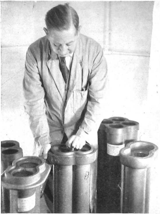
Fig. 3 : Gauging the socket of a self-aligning duct
