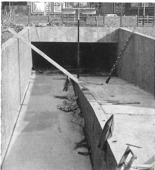
Fig. 3 (above) : Subway being constructed
