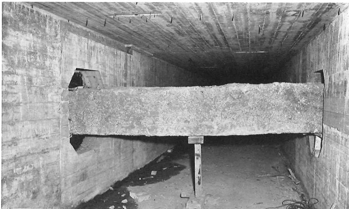
Fig. 4 (below) : 9-way duct, with cables still working, surrounded by concrete
