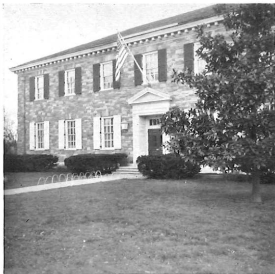
A Central Office (Telephone Exchange) at Washington, D.C.
