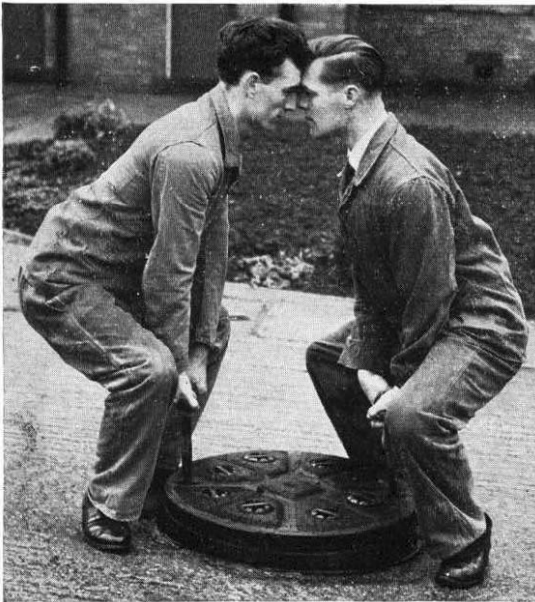
Lifting a heavy manhole cover
