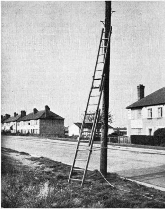
Fig. 5 : Extension Ladder lashed to pole
