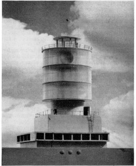
Radio relay stations of the future operating on centimetric wavelengths will look like this. Microwave links will replace multiple aerial arrays
