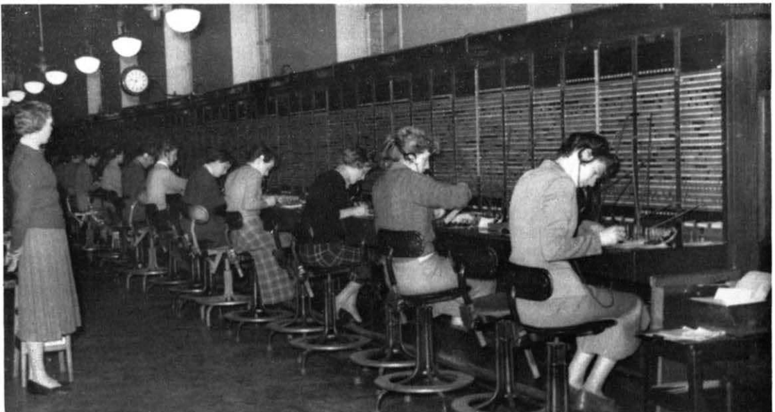
A junior team at the switchboard
