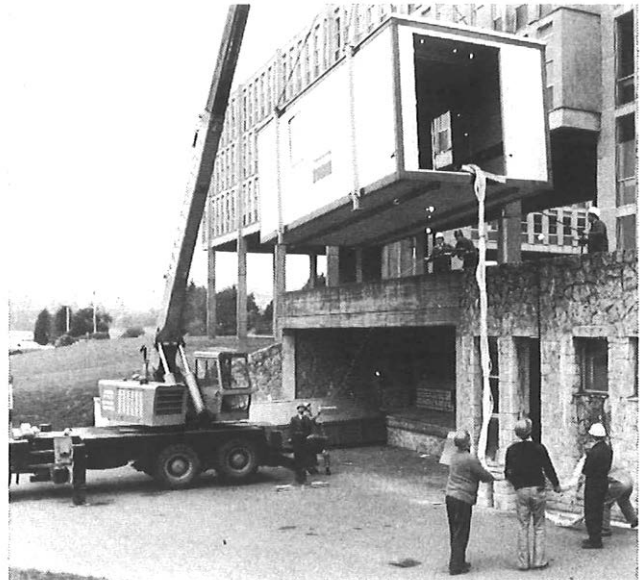
FIG. 3—The Portakabin being hoisted into position
