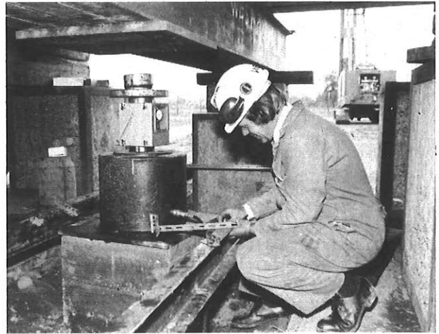
FIG. 11—Pile testing showing jack positioned between pile and kentledge
