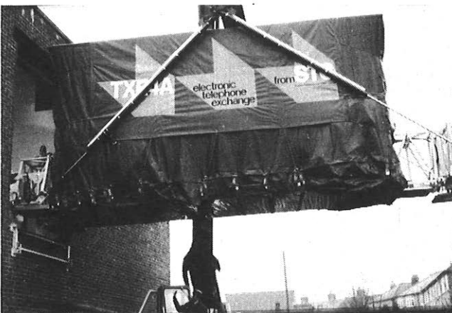
FIG. 2—Largest module being manoeuvred by telehoist
