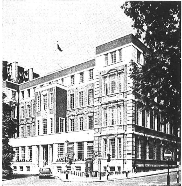
FIG. 2—The IEE building, Savoy Place, London
