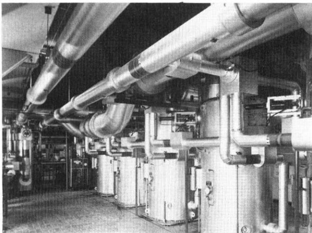
FIG. 9—Waste-heat boilers
