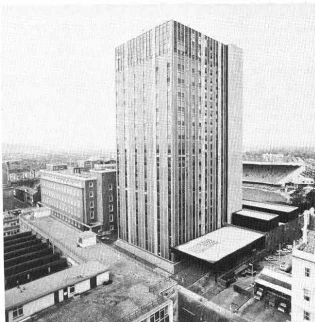
FIG. 1—Cardiff telephone exchange
