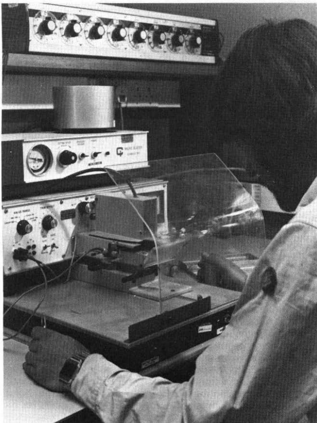
FIG. 5—Adjusting resistors by air-abrasive trimming
