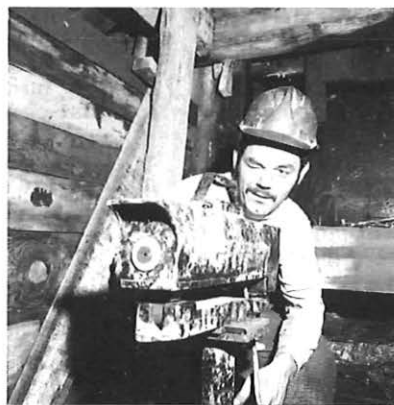
FIG. 3—Aligning the laser
