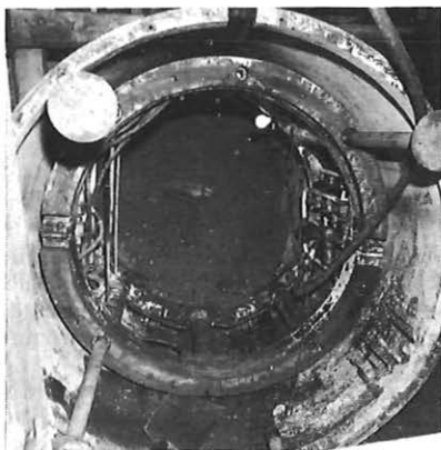
FIG. 2—Shield, showing driving rams
