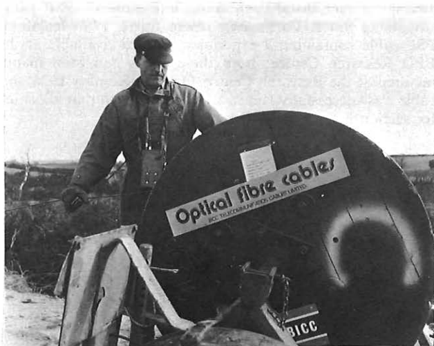
FIG. 4—Cable installation by Colchester Telephone Area staff
