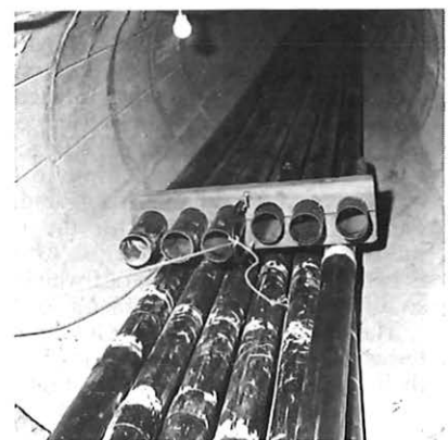
FIG. 4—The 6-way pulling clamp
