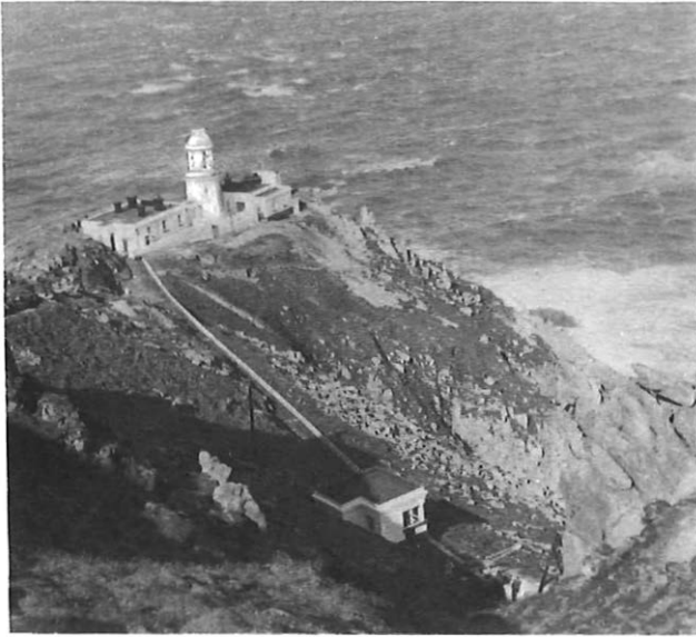
FIG. 3—The northern lighthouse
