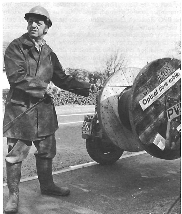
FIG. 8—Installation by Colchester Area staff of optical-fibre cable
