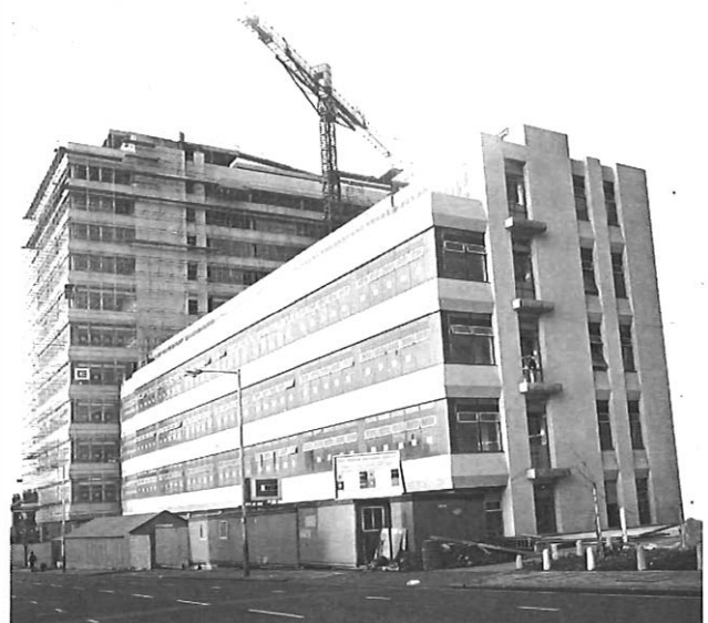
Ilford SSC under construction in 1971
