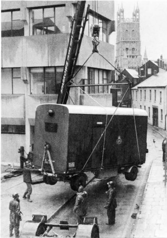
FIG. 3—Mobile unit 7 being removed from the compound
