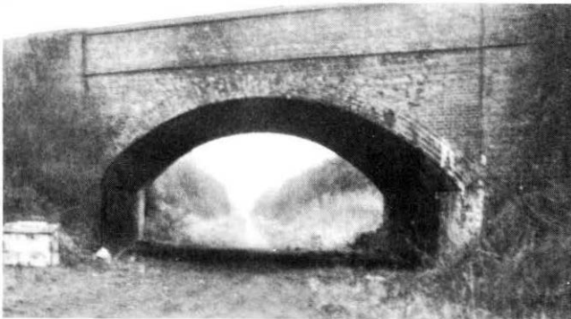
FIG. 1—The bridge before demolition, viewed from the level of the old railway track
