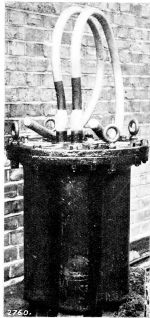
5.—LOADING COIL CASE.
