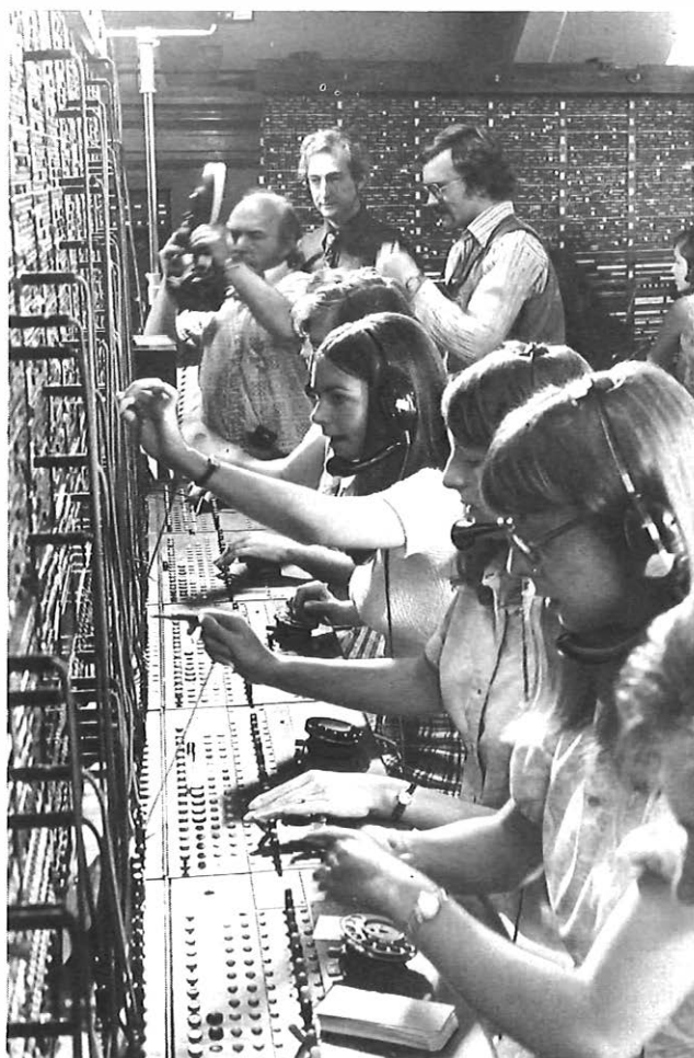
FIG. 1—Face panels at Braintree CB 10 before conversion
