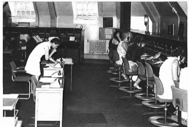
Fig. 4—General view of Braintree AMC after conversion, showing the main and island suites, and modern equipment tables
