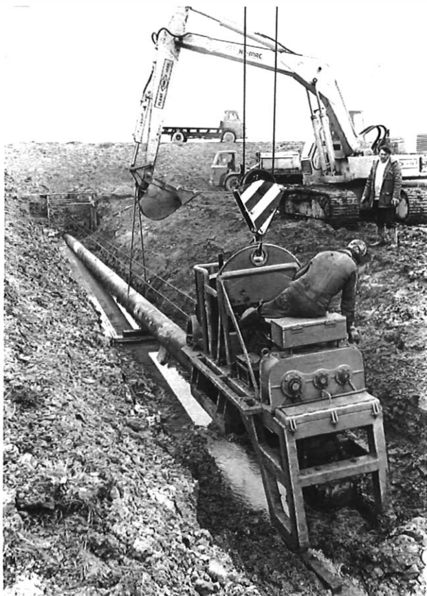
FIG. 2—The auger borer in operation
