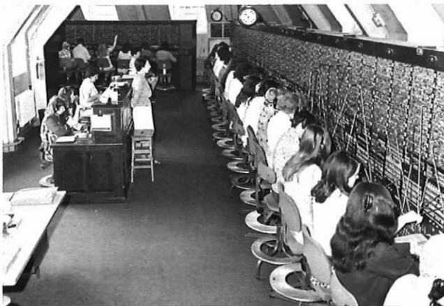
Fig. 3—General view of Braintree CB 10 before conversion, showing the main suite (right), the island suite (background), and the enquiry suite and supervisor's console (left)
