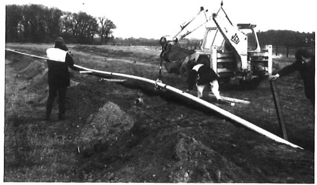
FIG. 8—Duct being placed in trench by roller technique
