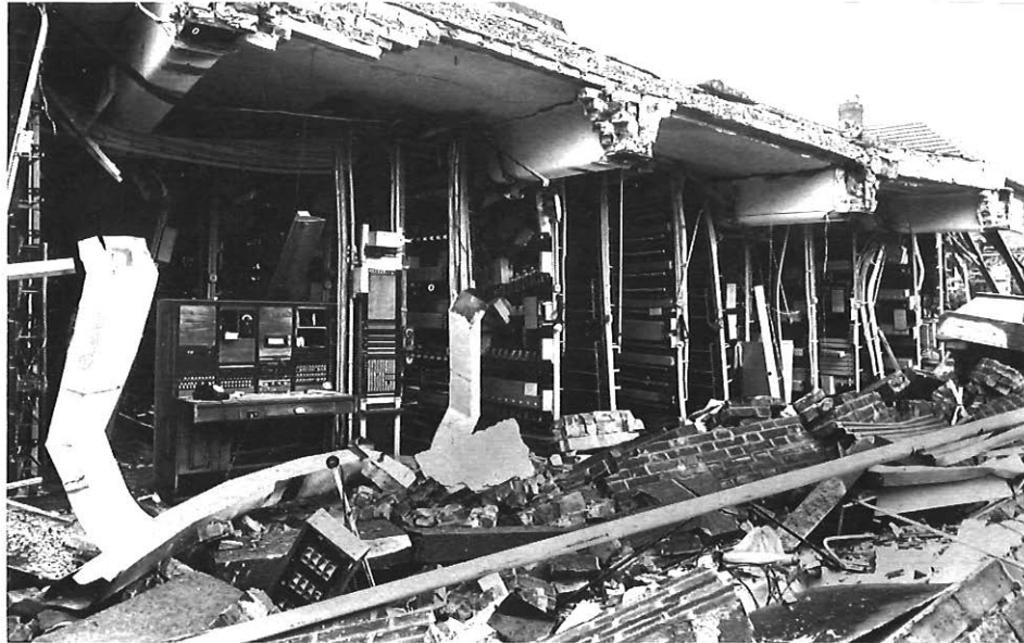
FIG. 2—Bishopwearmouth exchange after gas explosion
