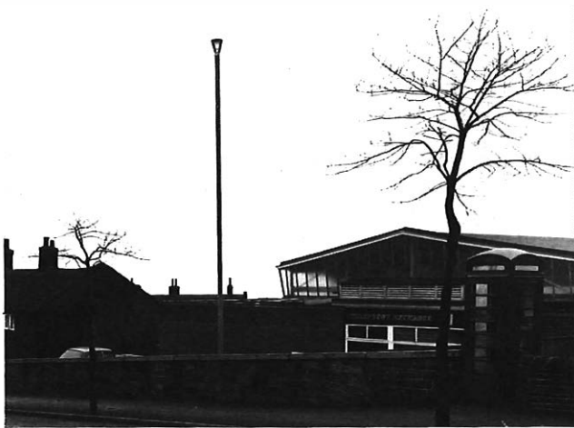
FIG. 4—Vent pipe at exchange manhole
