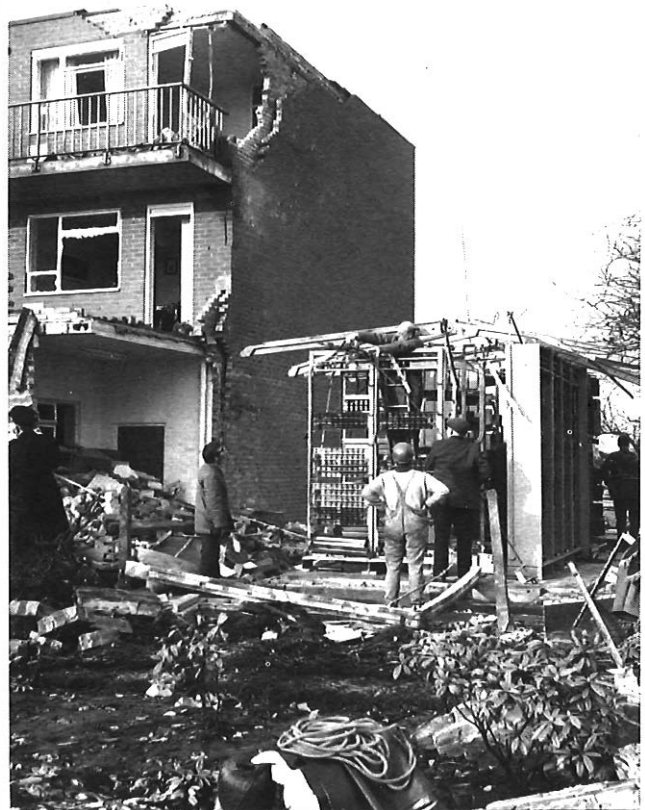
FIG. 1—Madeley exchange after gas explosion
