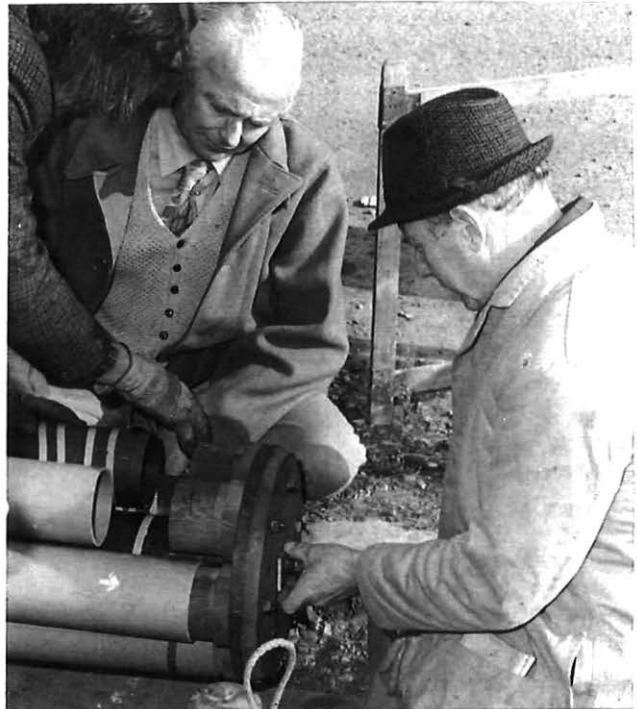
Fitting the front former to the ducts
