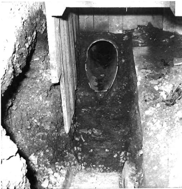
The gas pipe and duct-entry pit
