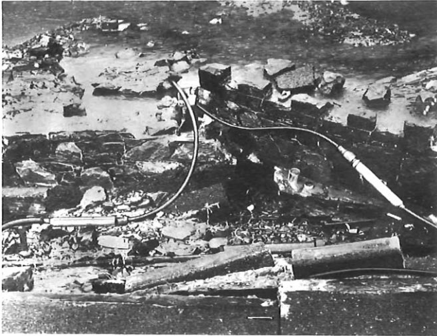
The exposed cables, showing the 3 m length of temporary repair cable jointed in
