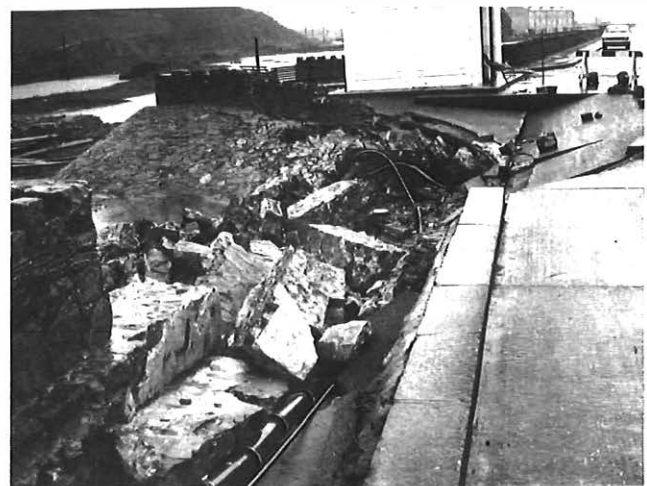
The collapsed sea front at Barmouth
