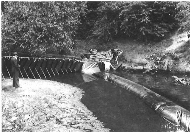
FIG. 2—Erection of the portable dam
