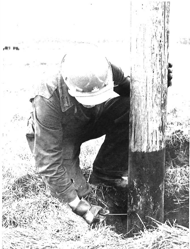
FIG. 2—Pole testing: inspection around the soil line
