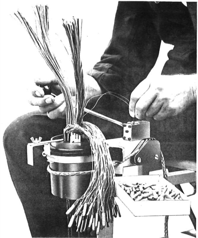
FIG. 13—Jointing jig in use with the Sleeve, Polyethylene No. 31A
