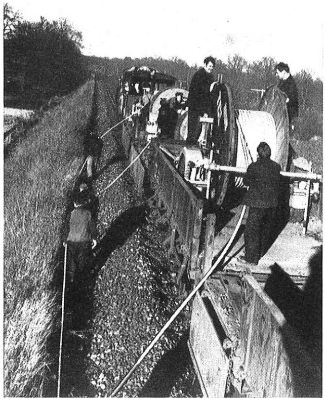
Simultaneous dispensation of three cables from the hired train.
