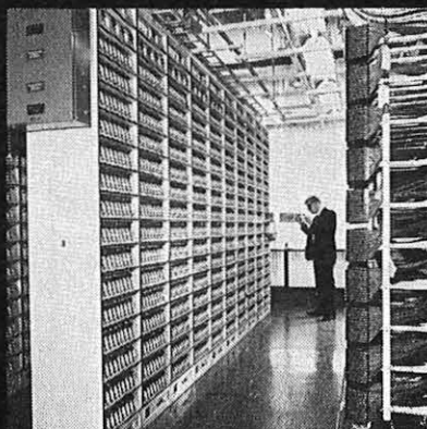
Telegraph Multiplex in London International Telex Exchange.
