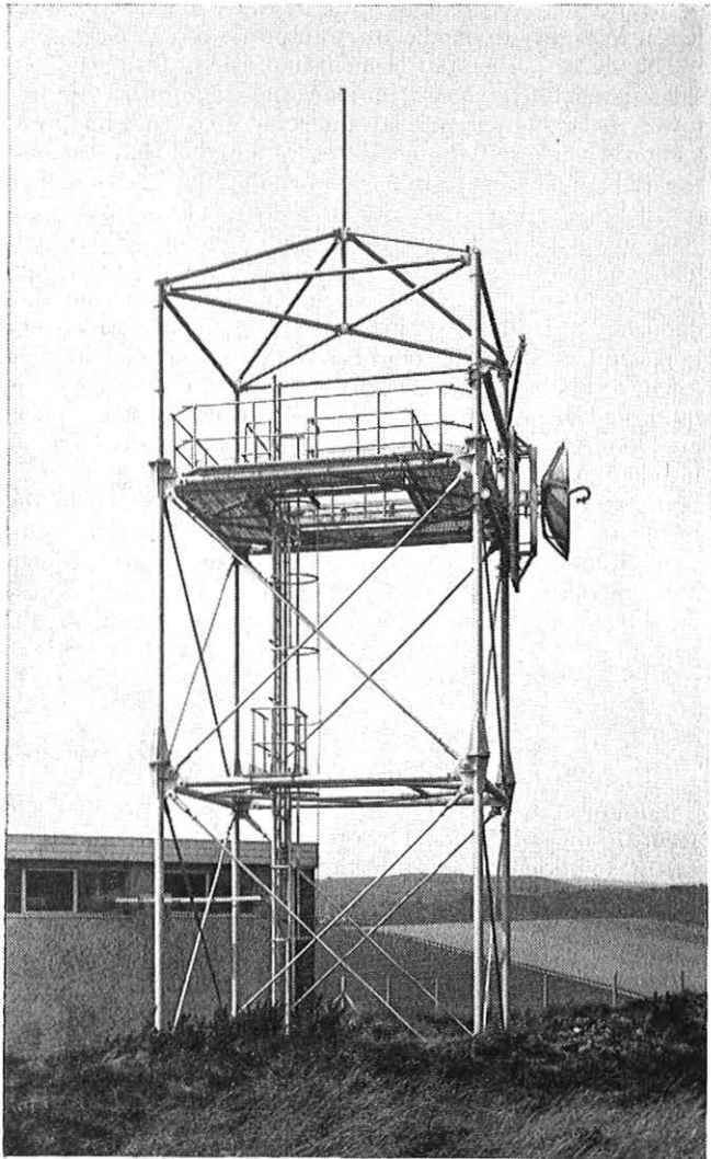
FIG. 18—A 45 ft high Tower No. 4A
