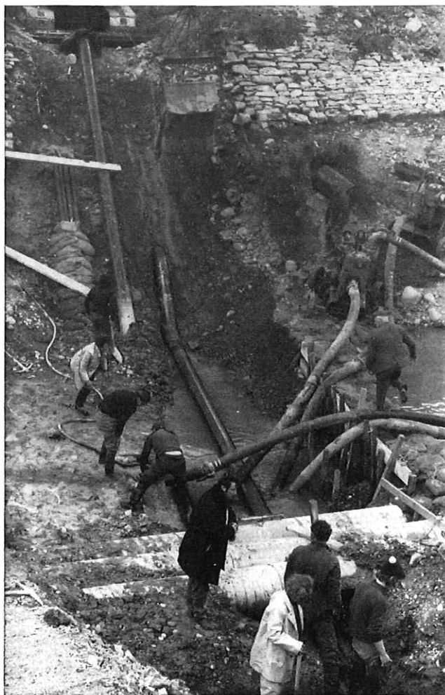
British Post Office duct with sand bag protection on the left and the other two services in position before reinstatement of canal bed and embankments.
