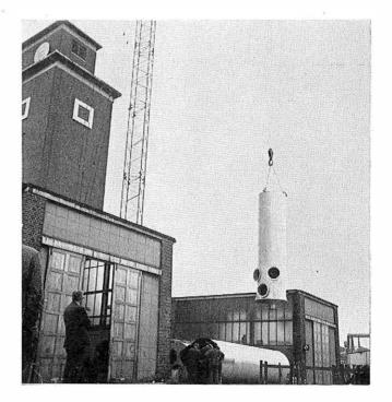
work was awarded to Thomas W. Ward Ltd. The three temporary chimneys were ready for use by January 1972 and had to be brought into operation at the end of April 1972 to allow an early start to the demolition work. The brick chimney was demolished in four weeks and the new chimney and flues were supplied, erected and the plant tested by mid-July.
