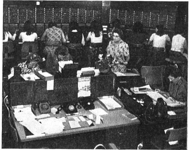
View of the Manual Exchange switch room during the last hours of its life
