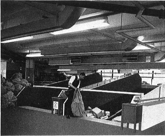
FIG. 4—Vertical riser discharge chute
