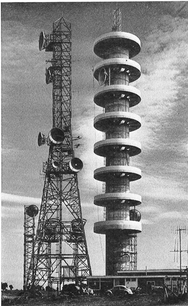
Fig. 3—Tower almost complete, with aerials mounted on first and sixth galleries
