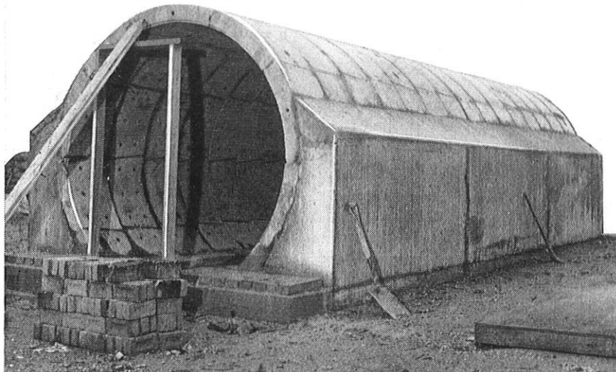
FIG. 1—Concrete tube constructed above ground for loading trials
