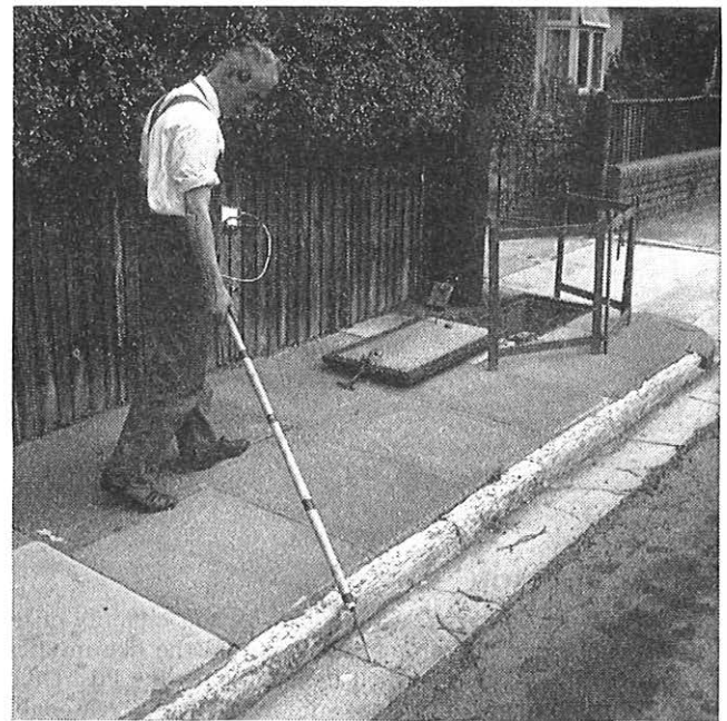
FIG. 5—The overground earth test using an experimental probe
