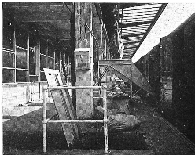
FIG. 1—Main rail platform
