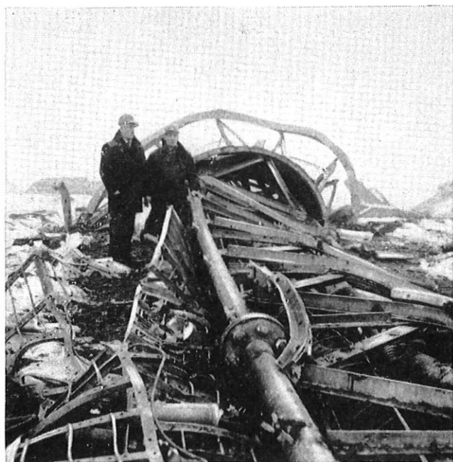
Wreckage of the main mast
