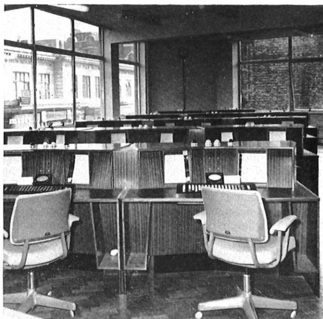
FIG. 3—Semi-automatic routing positions
