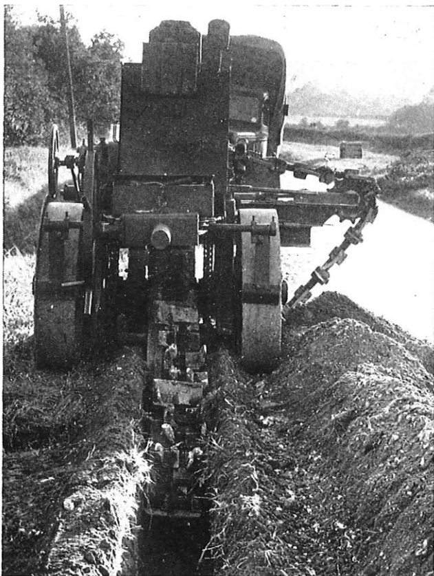
FIG. 1—AVELING-BARFORD TRENCH CUTTER
