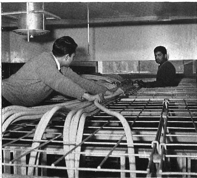
FIG. 5—CABLES BEING PLACED INTO POSITION ON THE GRID CABLE-PLATFORM
