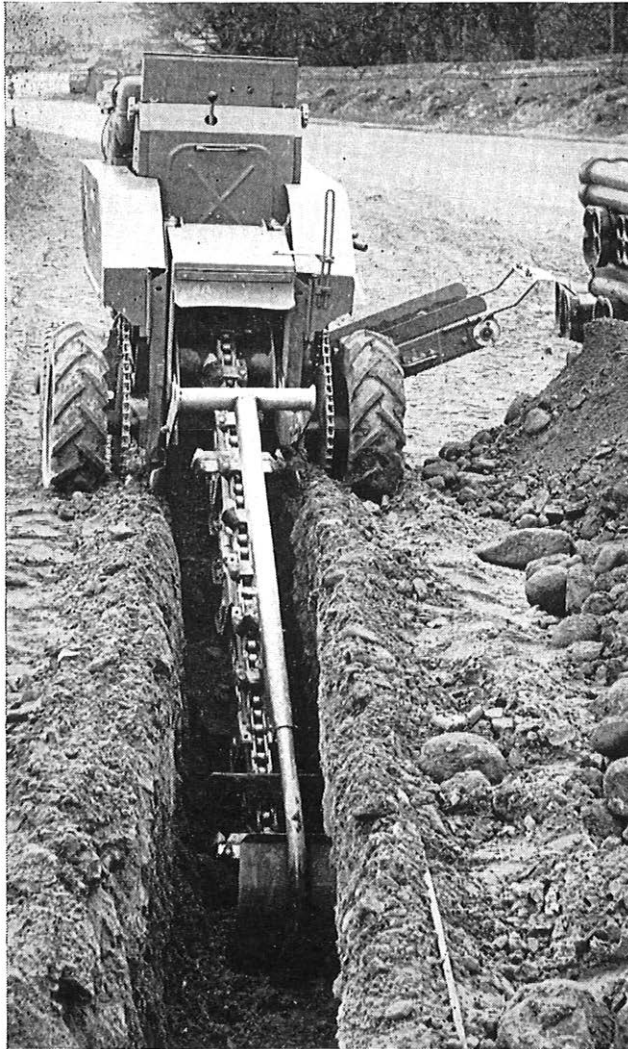
FIG. 5—TRENCH EXCAVATOR No. 2
