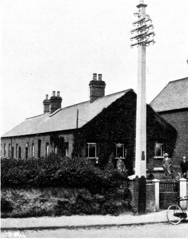
2.—NORTH WALSHAM REPEATER STATION.
