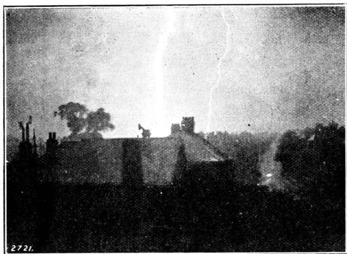
3.—THE CAUSE OF THE DAMAGE.
