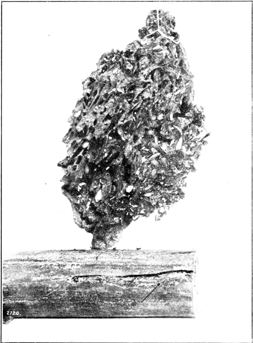
5.—A PIECE OF THE BUTT OF THE POLE ADJACENT TO DAMAGED DUCT.
