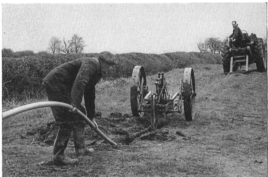
FIG. 7—CONTROLLING ANGLE OF DUCT ENTERING PIT
