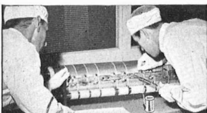
*Ersin Multicore Solder is shown being used at the Brith factory of Submarine Cables Ltd., in the production of a submersible repeater designed to last for a minimum of 20 years under the sea without attention.*
