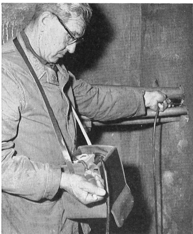
FIG. 2—TESTING FOR GAS AT A DUCT MOUTH
