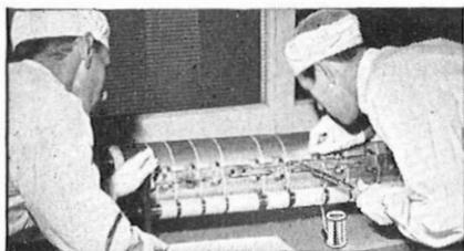
*Ersin Multicore Solder is shown being used at the Erith factory of Submarine Cables Ltd., in the production of a submersible repeater designed to last for a minimum of 20 years under the sea without attention.*
