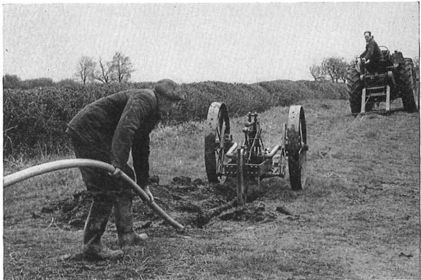
FIG. 7—CONTROLLING ANGLE OF DUCT ENTERING PIT
