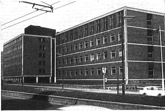
HUDDERSFIELD NEW AUTOMATIC TELEPHONE EXCHANGE
