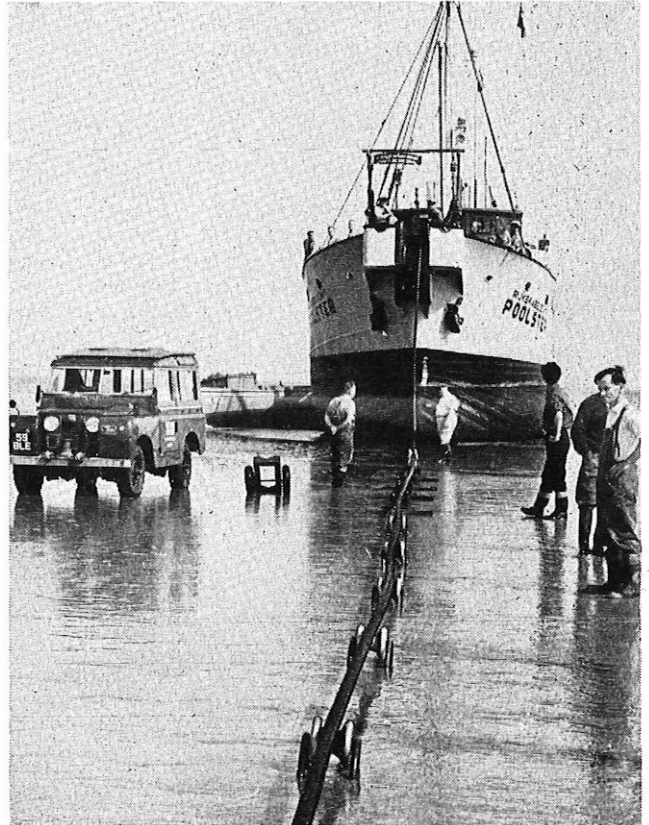
CABLE BEING HAULED ASHORE FROM POOLSTER
