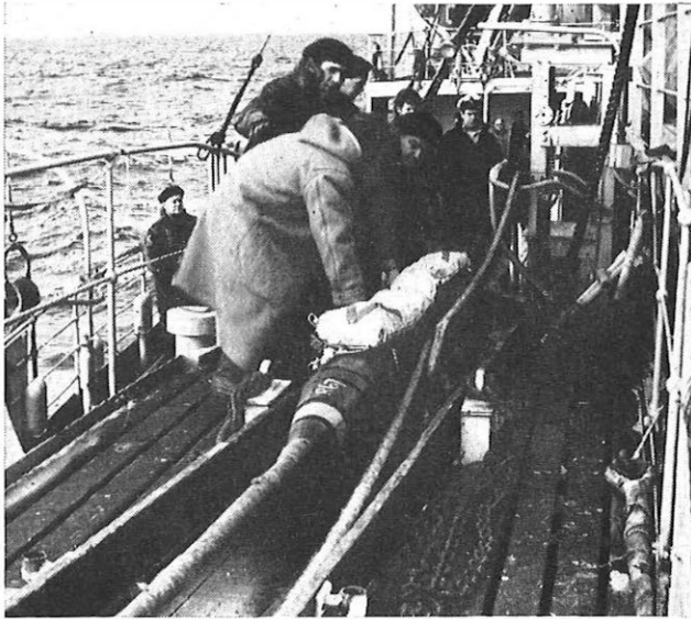
FIG. 5—LAUNCHING A REPEATER WITH PARACHUTE
