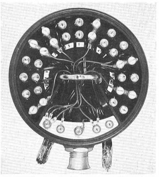
THE MODIFIED BLOCK TERMINAL SHOWING PROTECTORS FITED TO SIX LINES
