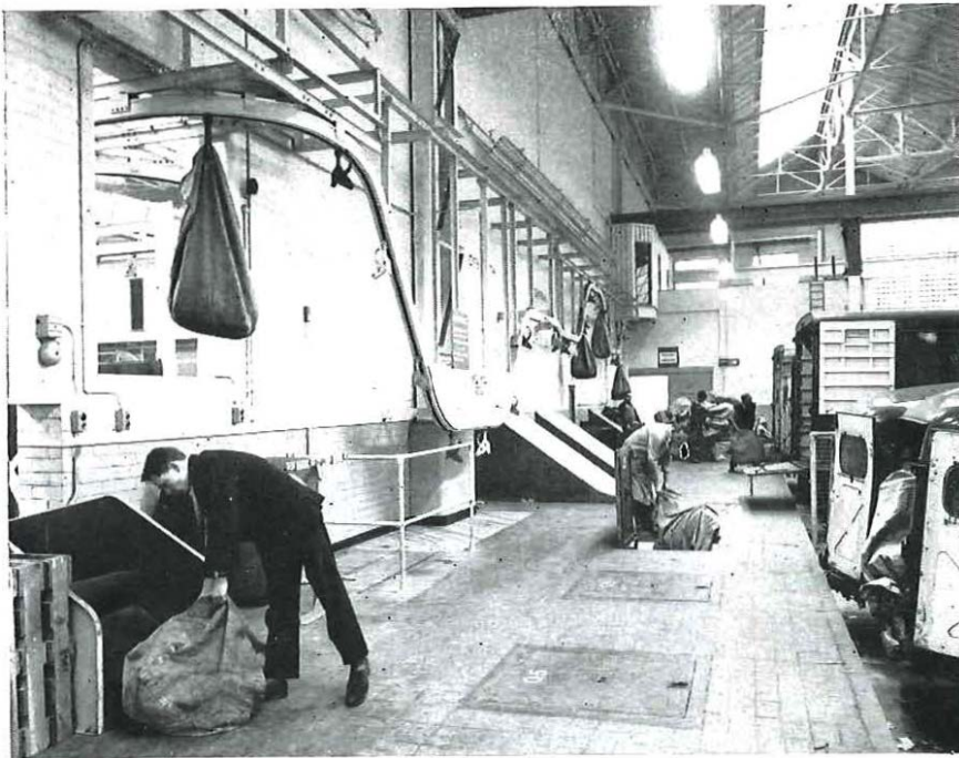
FIG. 3—LOADING PLATFORM SHOWING THE CHAIN CONVEYOR AND THE FLOOR LOADING TRAPS
