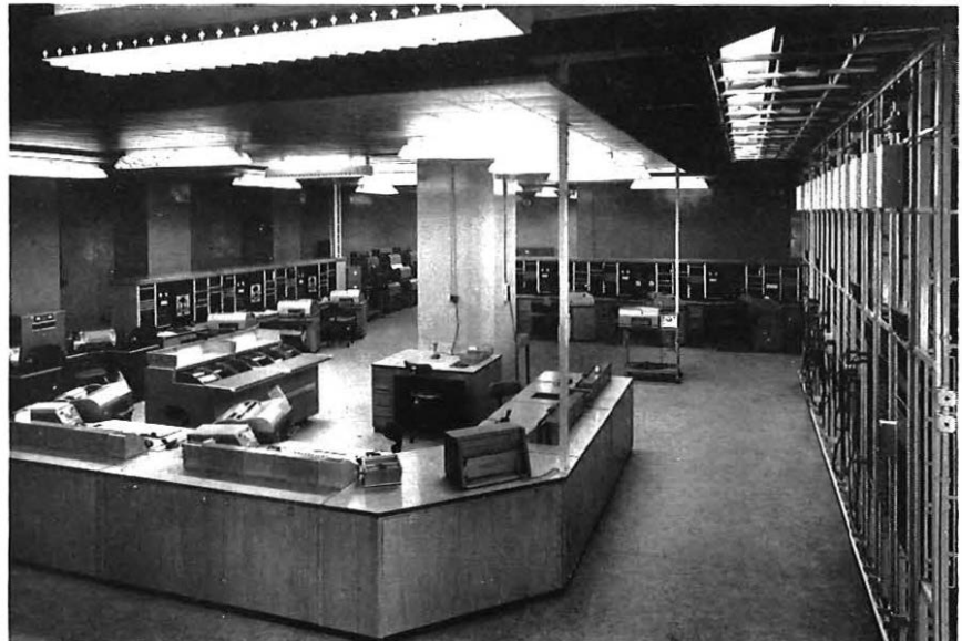
In the foreground are maintenance-control positions.
