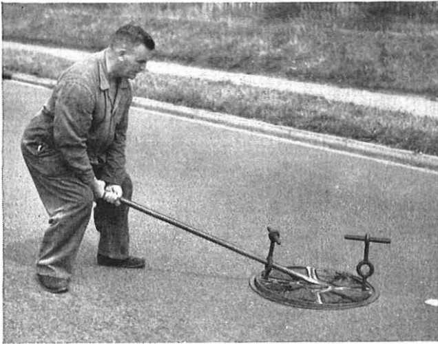
FIG. 7—EASING A MANHOLE COVER USING A CROWBAR
