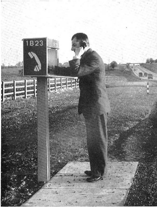
FIG. 4—GENERAL VIEW OF ROADSIDE TELEPHONE
