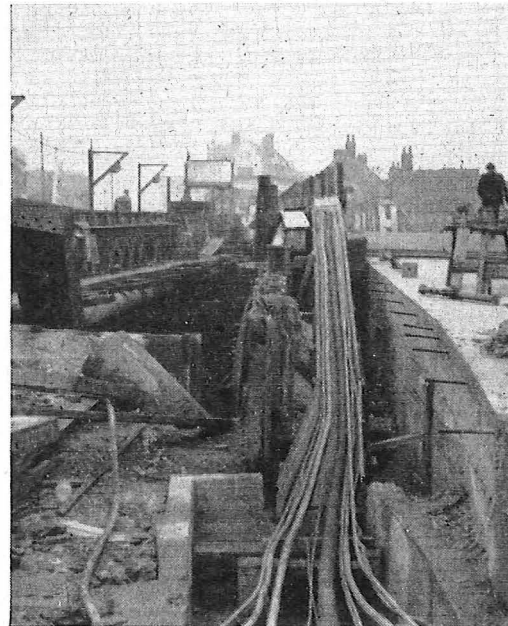
RECONSTRUCTION OF MILL BRIDGE, DONCASTER
