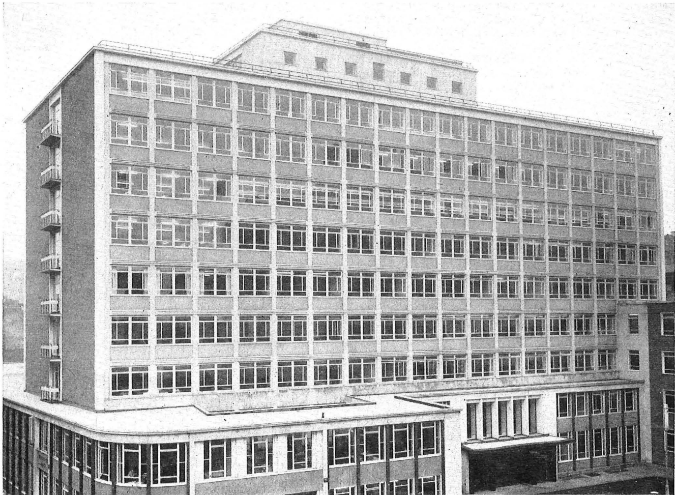
2-12 GRESHAM STREET, LONDON, E.C.2
