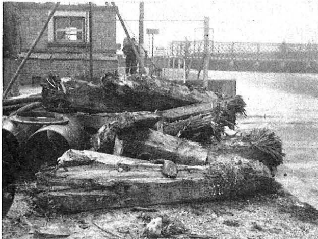
FIG. 8—OLD PILES DREDGED FROM HARBOUR BED
