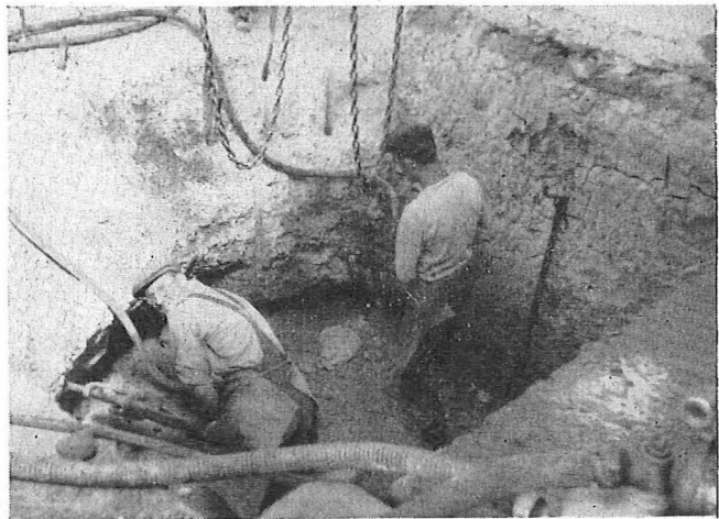
BREAKING UP THE OLD FOUNDATIONS
