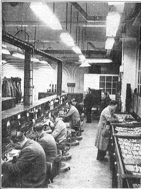
FIG. 9.—ILLUMINATION OF TEST DESKS BY FLUORESCENT LIGHTING.
