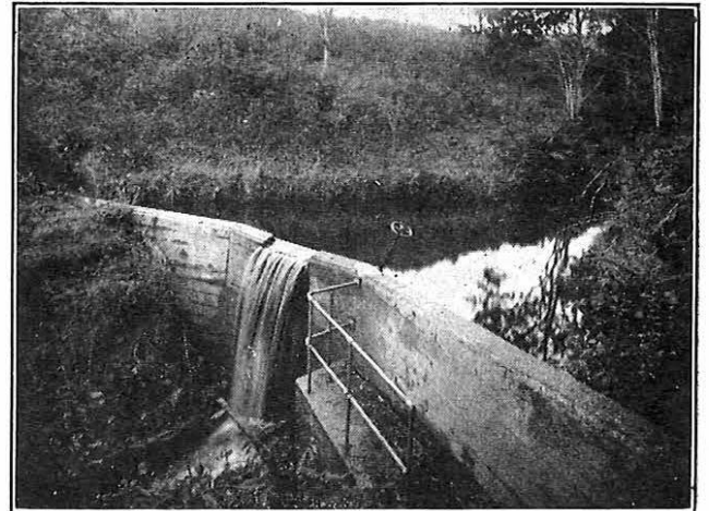
FIG. 17.—POND USED FOR ENGINE-COOLING WATER.
