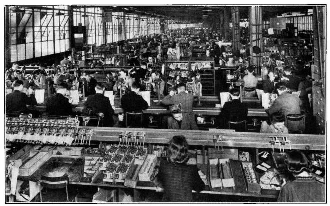
MAIN ASSEMBLY AND WIRING OF 2,000-TYPE SELECTORS.
