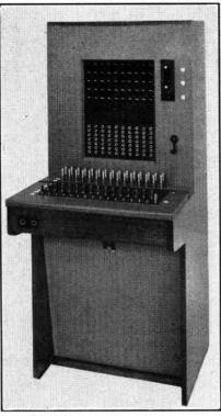
FIG. 17.-MODERN CORD SWITCHBOARD.
