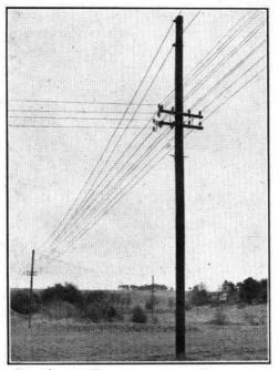
FIG. 18.—AN ENAMPLE OF JOINT TELEPHONE AND LOW-VOLTAGE POWER-LINE CONSTRUCTION.
