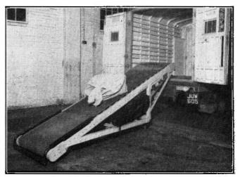
FIG. 2.—VEHICLE-LOADING CONVEYOR.
