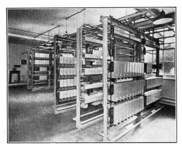
FIG. 21.—Typical 500-Line Installation of P.A.B.X. No. 3.
