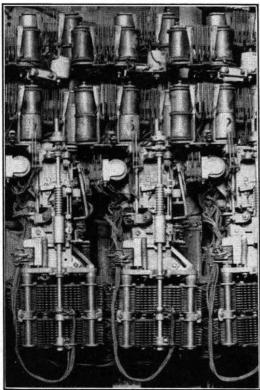
FIG. 4.—FINAL SELECTORS AT EPSOM EXCHANGE, 1912.
