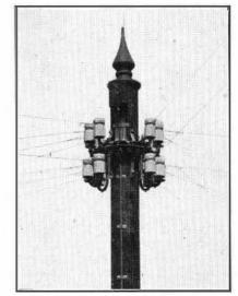
FIG. 5.—THE TOP OF A RING-TYPE DISTRIBUTION POLE.
