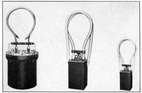
1<u>12 inches</u> Note: Left to right, 1924-1931, 1931-1951, after 1951. FIG. **11**.---TYPICAL LOADING POTS, EACH CONTAINING 108 LOADING COILS.
