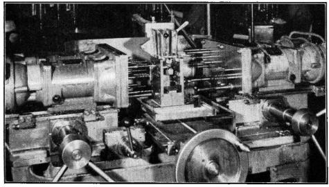
MULTIPLE-SPINDLE DRILLING MACHINE FOR 2,000-TYPE SELECTOR FRAMES.
