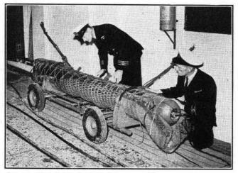
FIG. 3.—THE FIRST BRITISH SUBMARINE TELEGRAPH REPEATER.
