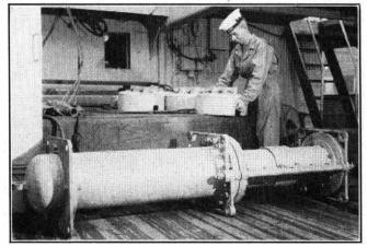
FIG. 8.—SHALLOW-WATER SUBMARINE TELEPHONE REPEATER.
