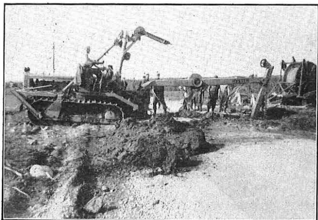
FIG. 11.—ONE OF THE TRENCHING MACHINES AT WORK.
