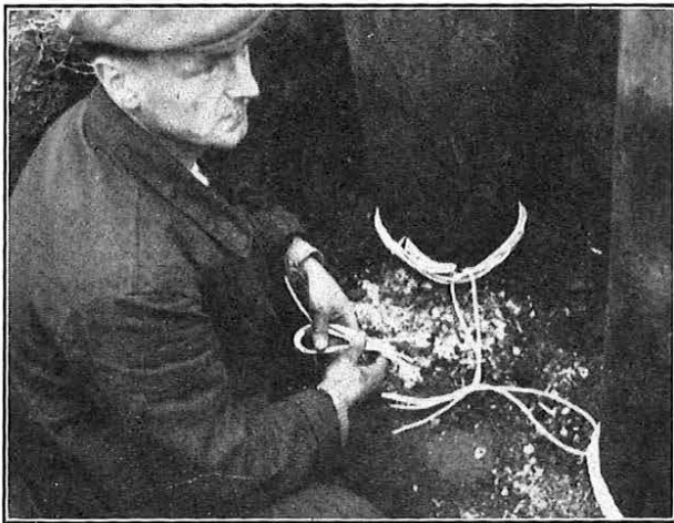
ATTACHING THE DETONATING FUSE TO A POLE.
