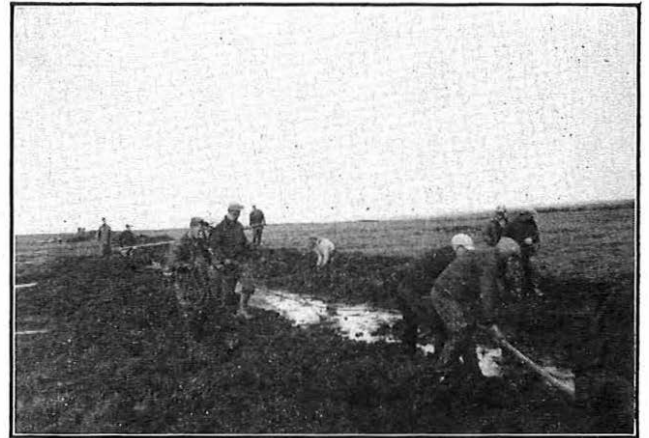
FIG. 13.—WORKING THE CABLE INTO THE TRENCH.
