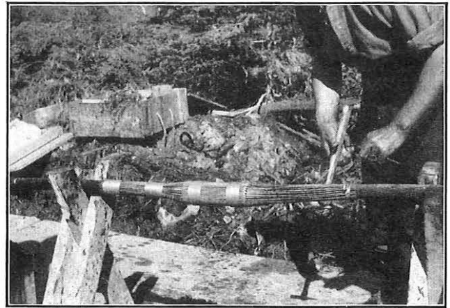
FIG. 20.—COMPLETING A SPLICE.
