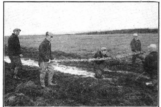
FIG. 14.—TREADING THE CABLE TO THE CORRECT DEPTH.
